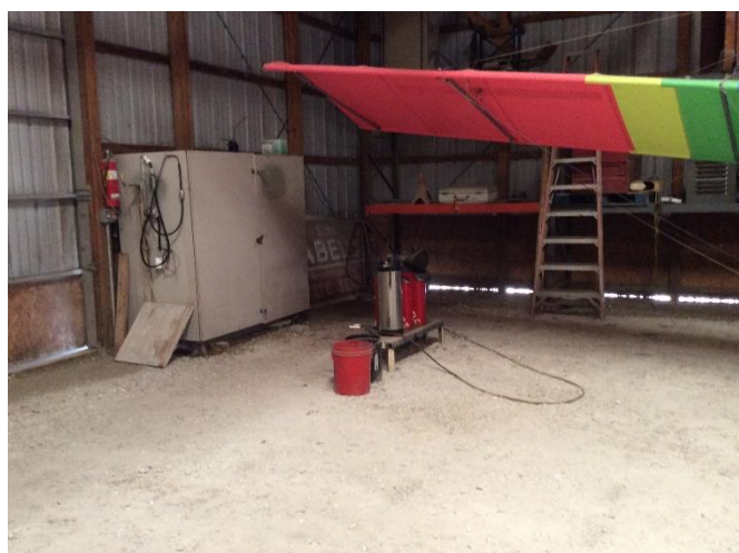
15. Additional gasoline canisters stored on pallets in the Pole Barn.
