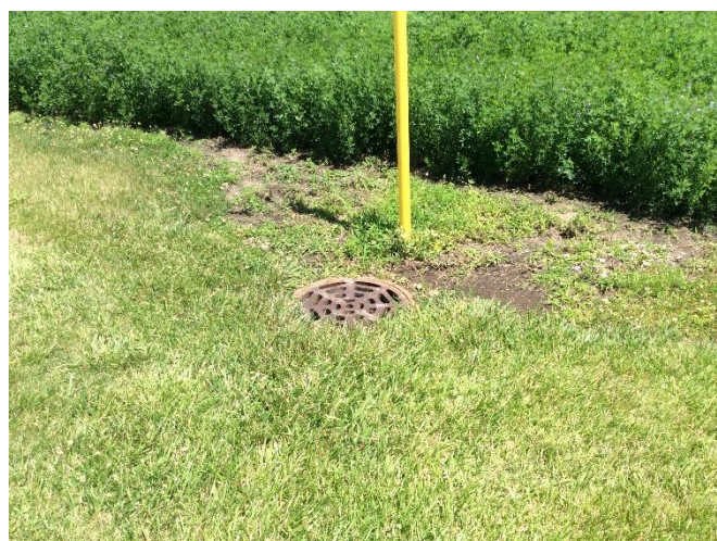
18. A stormwater drain located northeast of the Pole Barn.
