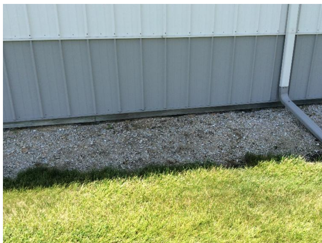
10. The Pole Barn is constructed atop a crushed stone foundation with a plastic interface.
